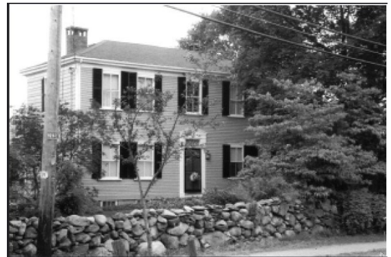
Stone wall in front of 300 Center Street. Owned & occupied by Abiel Edson in 1810. EHS
